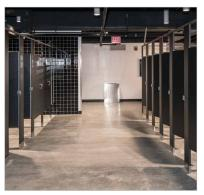
Durable Bradmar™ partitions are made from solid, one-inch thick HDPE (high density polyethylene) plastic that won't rust, delaminate, mildew or absorb odors.
